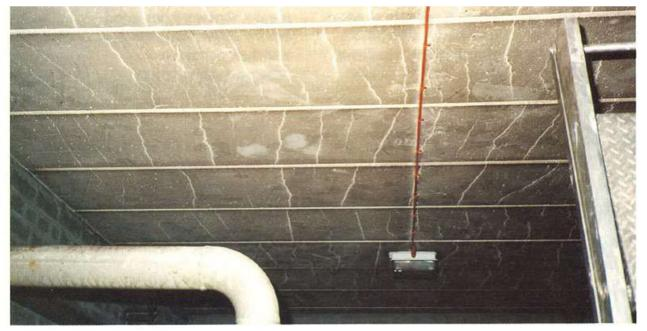
Figure 2 Widespread hair-line cracking on the soffits of many RAAC planks
